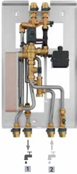
Fig. 15: Filling the potable water circuit
